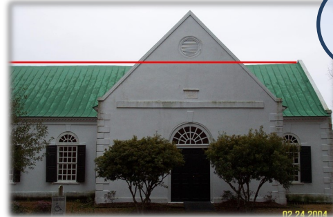
Left and right, off plumb walls and roof, courtesy of Richard Marks Restorations and Old St. Andrew's; center, view of the outward leaning south nave wall from the crossing of the aisles, photo by the author.
