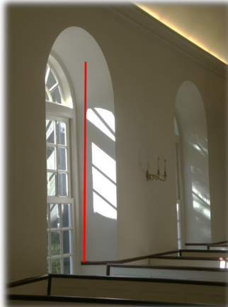
Left and right, off plumb walls and roof, courtesy of Richard Marks Restorations and Old St. Andrew's; center, view of the outward leaning south nave wall from the crossing of the aisles, photo by the author.
