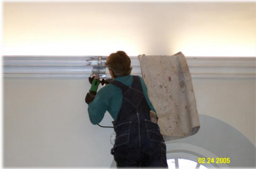
Top: Repairing the gutter for the cove lighting.
