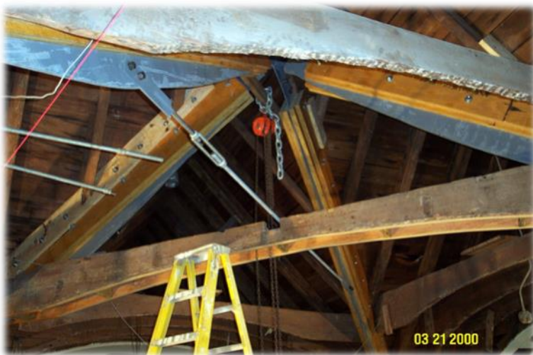
New steel and wood roof truss at the crossing of the aisles.
