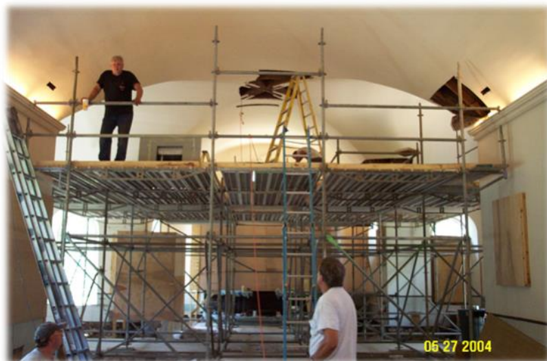
Revealing the valley rafters in the barrel vaulted ceiling.
