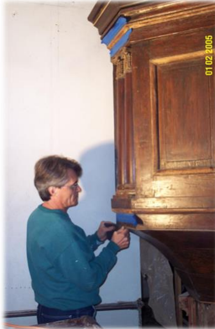
Pulpit repair, including fixing termite damage to the base and adding bolts to affix the top to the wall.
