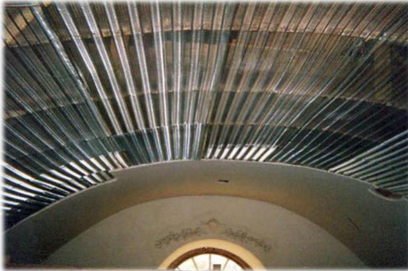
New steel lath ready for replastering.
