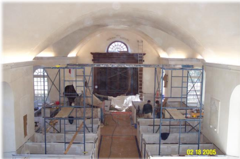
Replastering and repainting of the interior is nearly completed.
