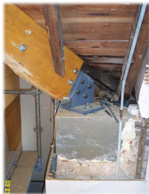
New roof truss base.
