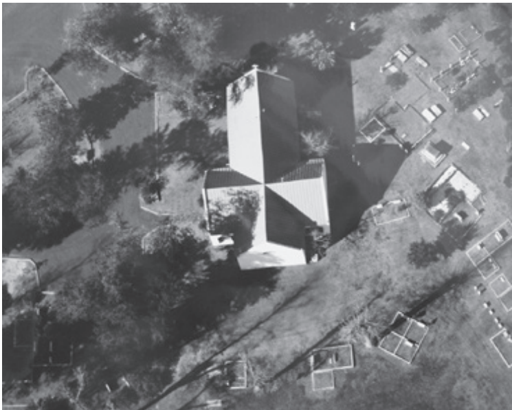
Aerial view of the cruciform church (Courtesy of St. Andrew's Parish Church)
