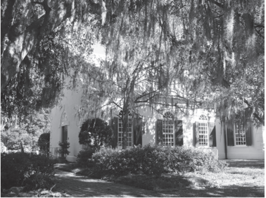
Church exterior, southwest elevation (Photo by the author)
