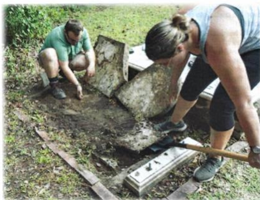
Grave of Mary C. Roach, students removing concrete poured inside the brick lining.
